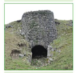
It was filled from the top with fuel and limestone and the burnt lime was taken out from the arched draw-hole below. Burnt lime has many potential uses but in this case it would have been spread on the fields to improve the soil.
