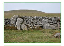
We can tell this is an older wall because the stones are irregular in shape with some large stones high up in the wall. This is characteristic of a wall built with stones cleared from a field rather than from quarried stone. In places there are also a number of large orthostats in the base of the wall.
